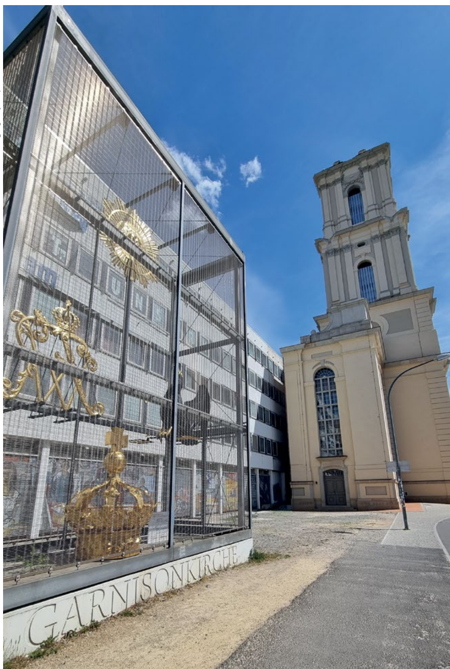
The 58-metre tower of the Garrison Church in Potsdam, rebuilt between 2017 and 2024 at a cost of over €44 million. In the future it will be crowned with a 30-metre spire bearing the already restored symbols of the Hohenzollerns (visible in the photo): the black Prussian eagle and the crown. A dispute continues over the reconstruction of the nave, where a computer centre building from 1971 is situated.
